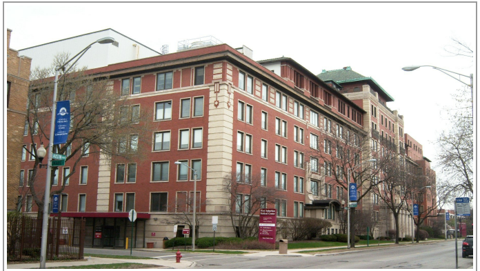
Original 1911 hospital building
