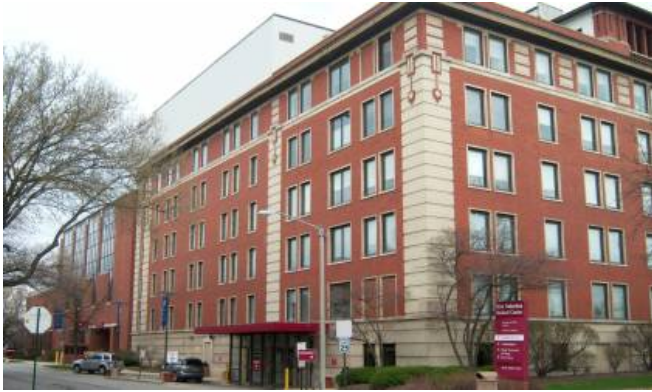
South addition (1922) and Pavilion (1996) on Ontario
