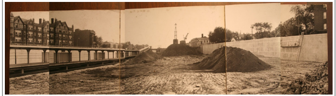
Photo taken during construction, ca. 1959-60
