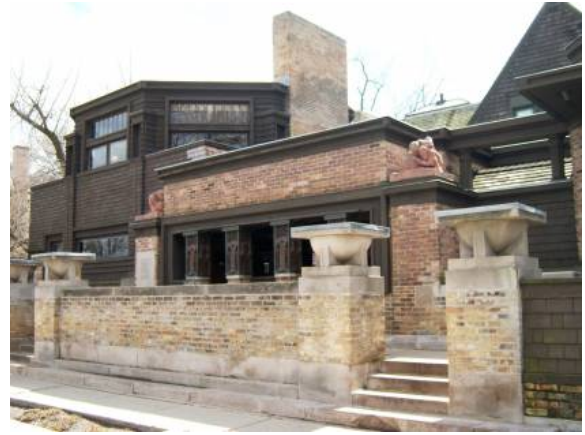
Studio facing Chicago Avenue (Village of Oak Park)
