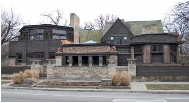
Studio facing Chicago Avenue (Village of Oak Park)
