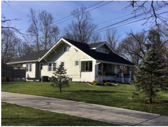
11829 E. 106th St., facing southwest. 2020
