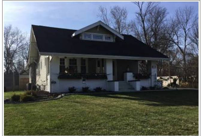
11829 E. 106th St., facing south. 2020
