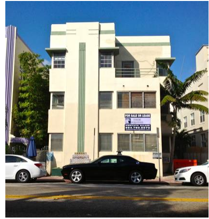
Wallack Apartments east elevation (view when facing west on Collins Avenue)
