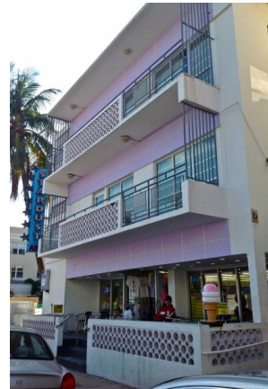
Primary facade of the Stardust Apartments
