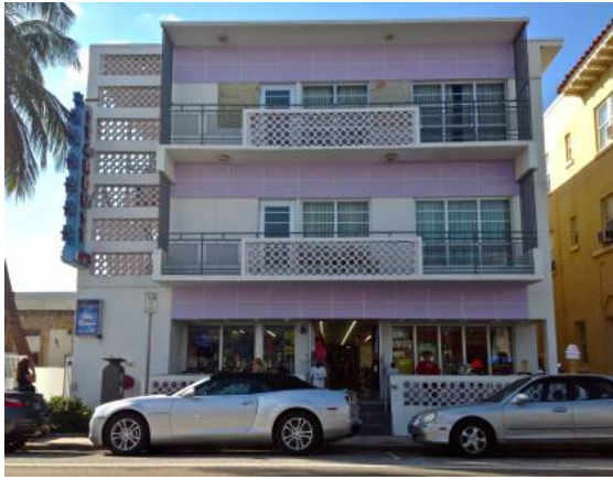
Stardust Apartments east elevation (view when facing west on Collins Avenue)
