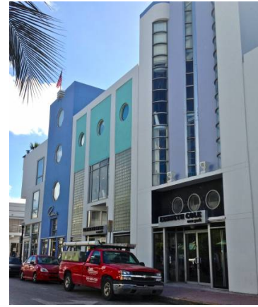
Detailed view of the north elevation of 763 Collins Avenue
