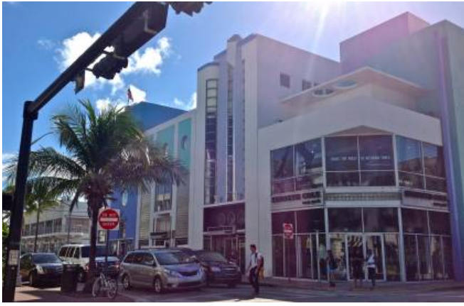
763 Collins Avenue north elevation (view when facing south on 8th street)
