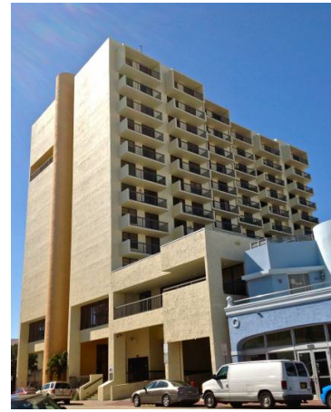
Northeast corner of Council Towers North
